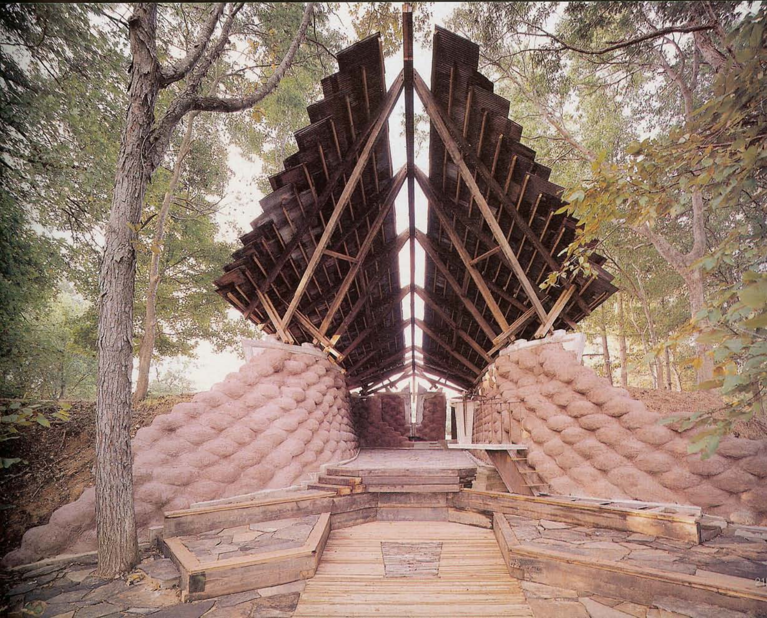
3 4 The rustic form of the chapel is inspired by vernacular farm buildings. 5 The great maw of the swooping roof, made from salvaged timber and tin shingles.
